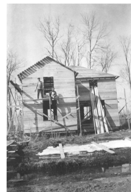
Charles Megarry house under construction
