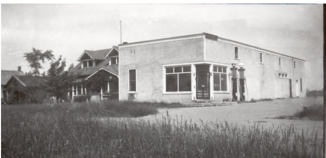
L to R: Harness shop, Wm. Megarry home, Megarry store. Stuccoed in the late 1930's.
